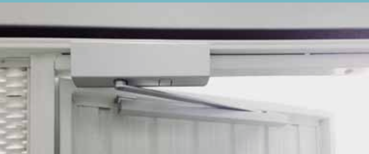
Overhead door closing mechanism with track.
