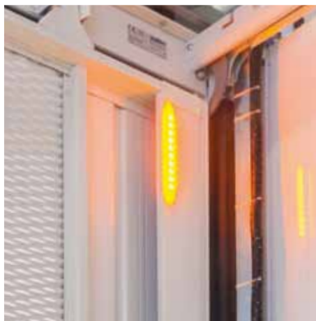
Internal flashing led unit, mounted and pre-wired.
