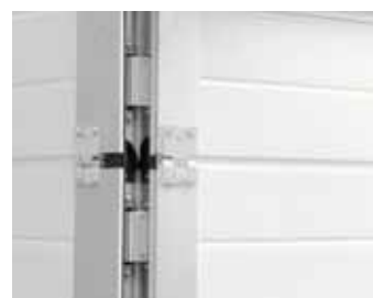
Detail of the concealed hinges of the pass door (inside view).
