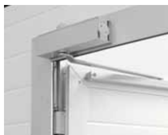
Detail of the overhead door closer mechanism of the pass door (inside view).
