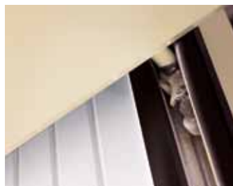
Anti-fall protection device incorporated in the tracks engages in the event of cable breakage, preventing the door leaf from dropping.
